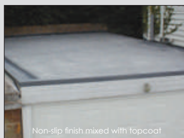
Non-slip finish applied onto topcoat with masked green detail
